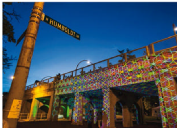
The new 606 elevated park connects four Chicago neighborhoods.
