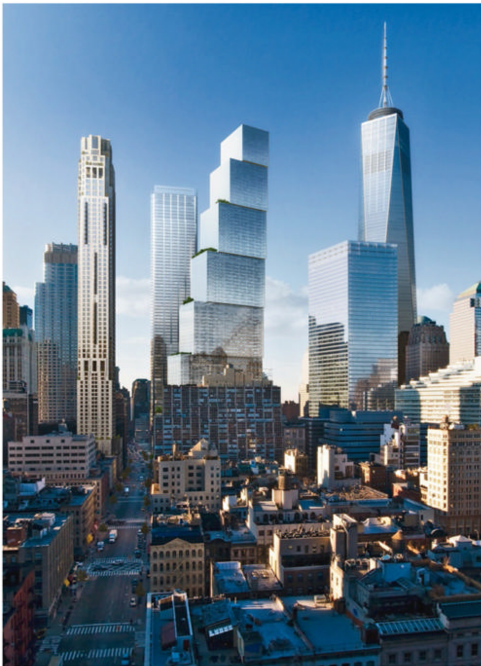
BIG’s design of 2 World Trade is made up of seven staggered boxes. Catered to a modern media company, each volume will function as its own building and include double-height atria, views between floors, and access to generous terraces.
